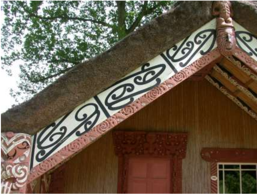
South maihi (bargeboard)
